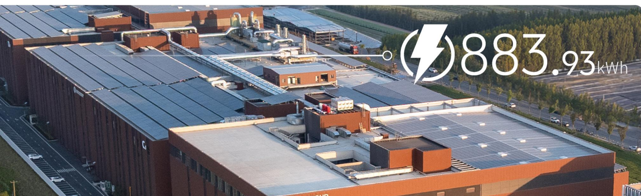
Total Power Generation of Shanghai Ailu in 2025 Reached 8,839,300 kWh.
